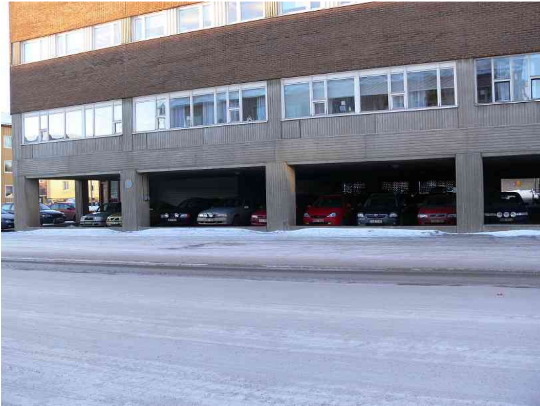
Photo 29 Luleo: parking on the ground floor of administrative building
