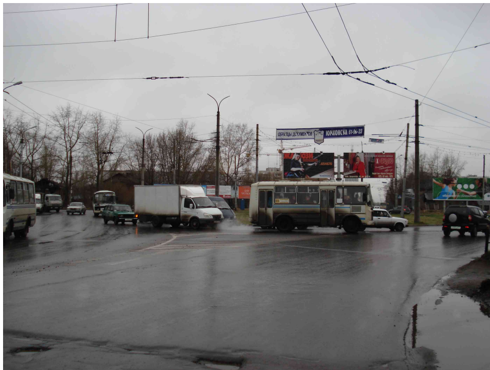
Photo Roundabout Voskresenskaya str/Obvodnyi Channel av.: wrong traffic organization – traffic is staying on the “ring”.
