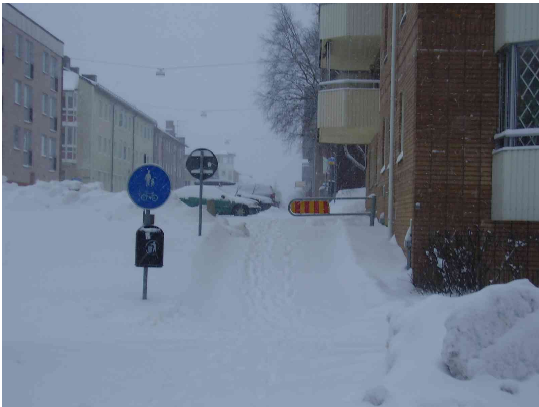
Photo 36 Luleo: barrier on the pedestrian and bicycle path
