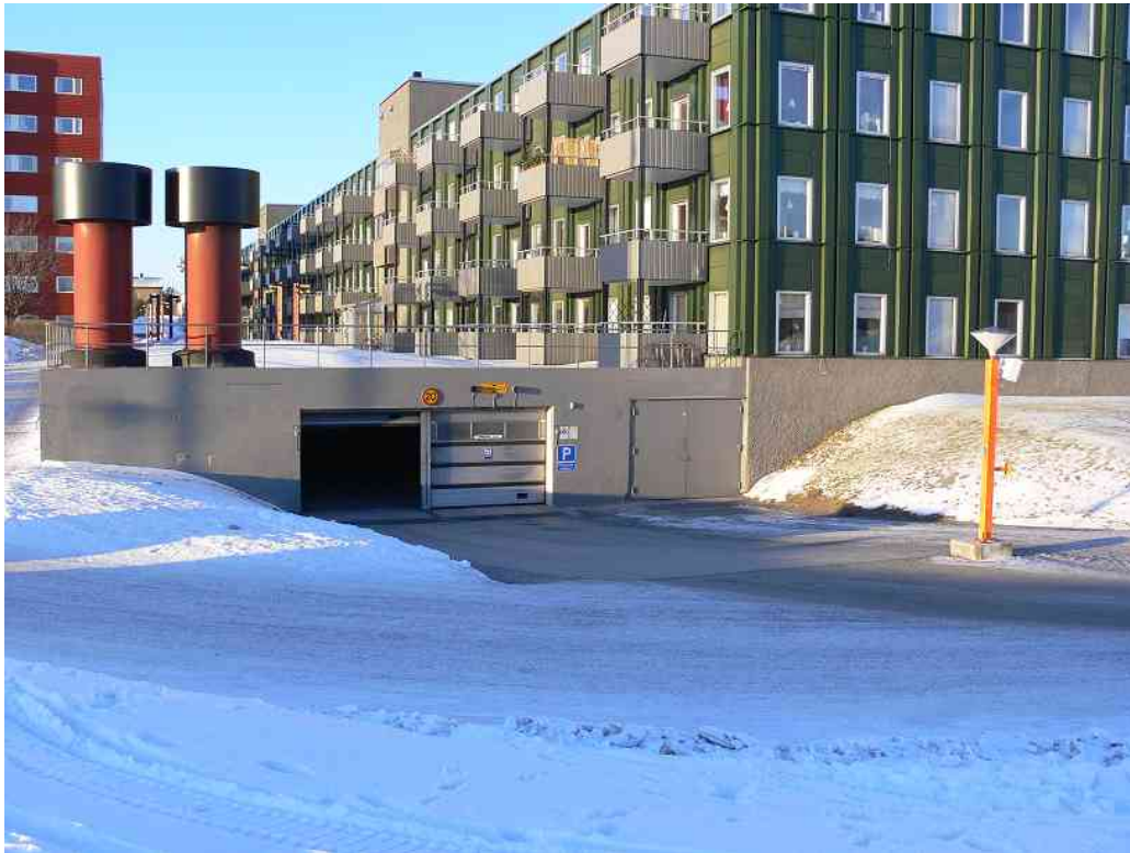
Photo 31 Luleo: underground parking
