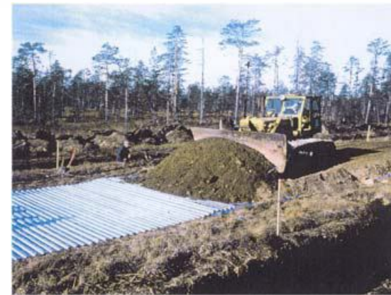
Narrow flange laid to the top Wide flange laid on the peatland surface
