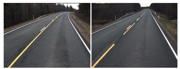
Figure 10. Section 505, direction 1: Left photo: 350 m. Differential frost heave related transverse cracks on side sloping ground. Right photo: 3200 m. Frost action related longitudinal cracking before the bridge.
