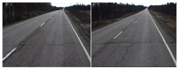
Figure 12. Section 515, direction 1: Left photo: 4000 m. Longitudinal, transverse and alligator cracking. Right photo: 4460 m. Longitudinal, transverse and alligator cracking.
