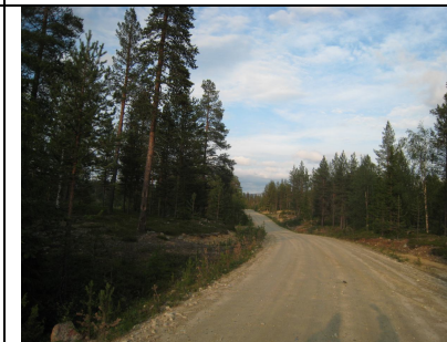
Photo 10 Example of a width-controlled gravel road
