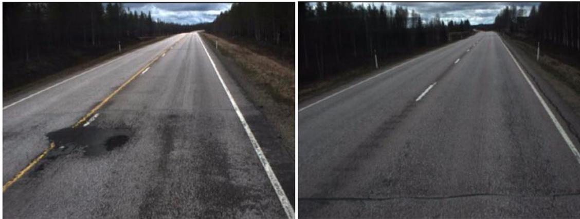
Figure 13. Section 515, direction 2: Left photo: 7000 m. Patch on the middle of the road. Right photo: 4360 m. Transverse cracking and left edge break.
