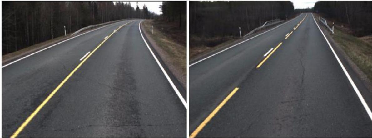
*Figure 10. Section 505, direction 1: Left photo: 350 m. Differential frost heave related transverse cracks on side sloping ground. Right photo: 3200 m. Frost action related longitudinal cracking before the bridge.*
