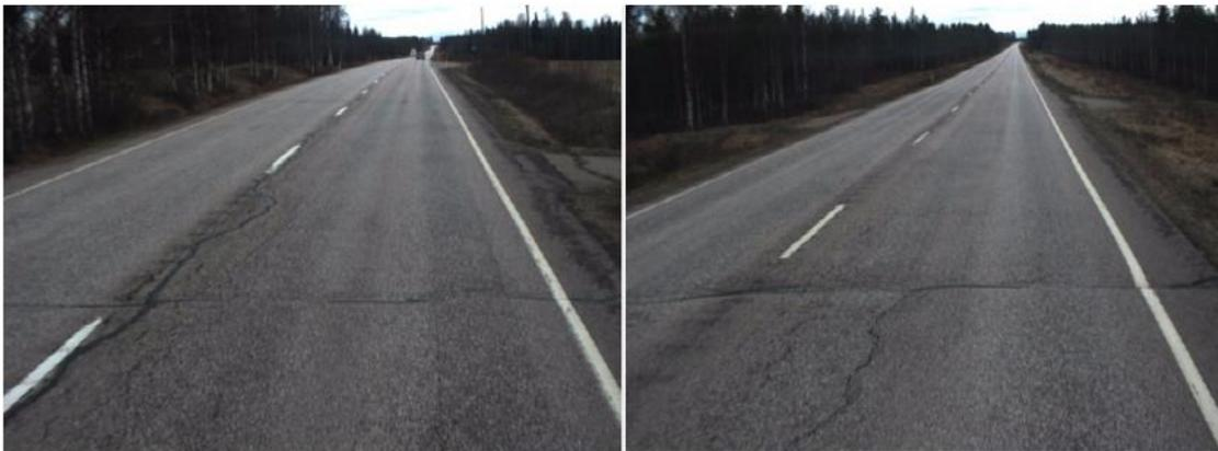
Figure 12. Section 515, direction 1: Left photo: 4000 m. Longitudinal, transverse and alligator cracking. Right photo: 4460 m. Longitudinal, transverse and alligator cracking.
